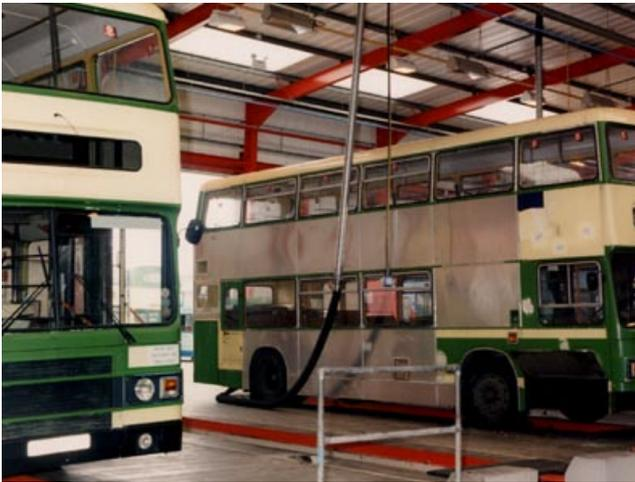
**Figure 3** Bus using a tailpipe exhaust extraction system to control emissions
